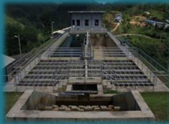
WATER TREATMENT PLANT AT AMBAGAMUWA GINIGATHHENA WSS
