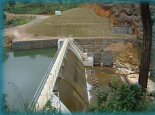
MOOL-OYA INTAKE, RIKILLAGASKADA WSS
