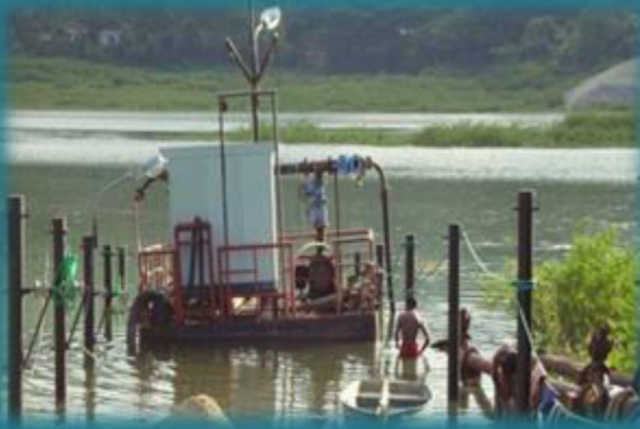
BALAGOLLA PONTOON INTAKE, KUNDASALE WSS
