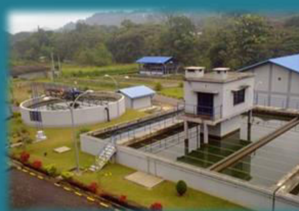
WATER TREATMENT PLANT AT MEEWATHURA, UDU-YATINUWARA WSS
