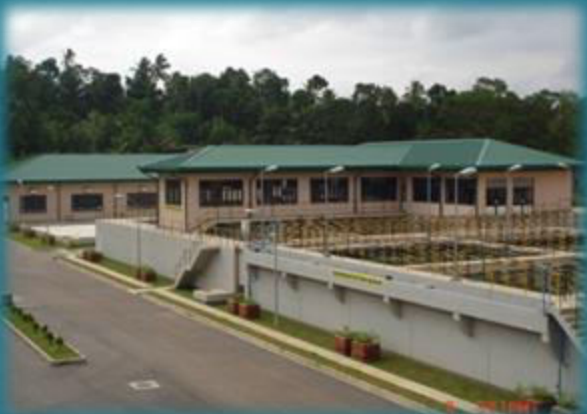
WATER TREATMENT PLANT AT KONDADENIYA, KATUGASTHOTA WSS
