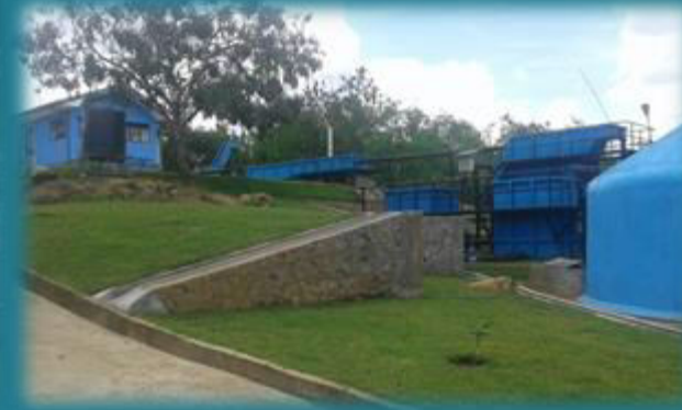
PACKAGE WATER TREATMENT PLANT AT WILGAMUWA FOR CKDU EFFECTED AREA
