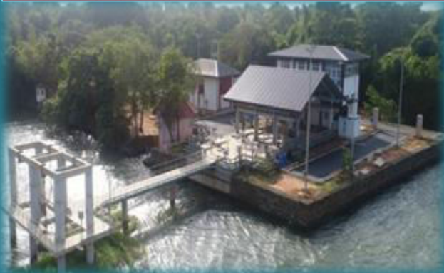
IBBANKATUWA RESERVOIR INTAKE, DAMBULLA WSS
