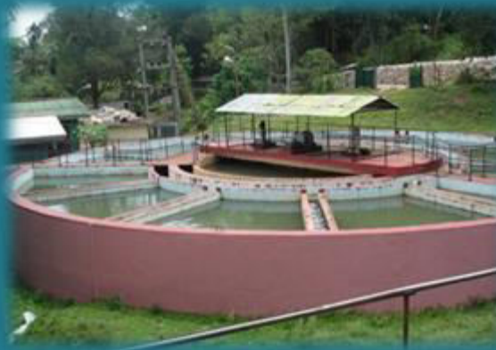
WATER TREATMENT PLANT AT MATHALE, MATHALE WSS
