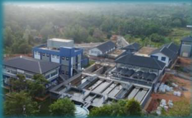
WATER TREATMENT PLANT AT DAMBULLA DAMBULLA WSS
